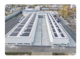
**GLS Germany:** the depot in Potsdam, Germany, is equipped with a photovoltaic system, which supplies electricity to the 70 charging points. Rainwater is collected on site and is used to irrigate the property. In September 2024, the building was awarded the Gold certification by the DGNB<sup>44</sup> for its sustainable building approach.
